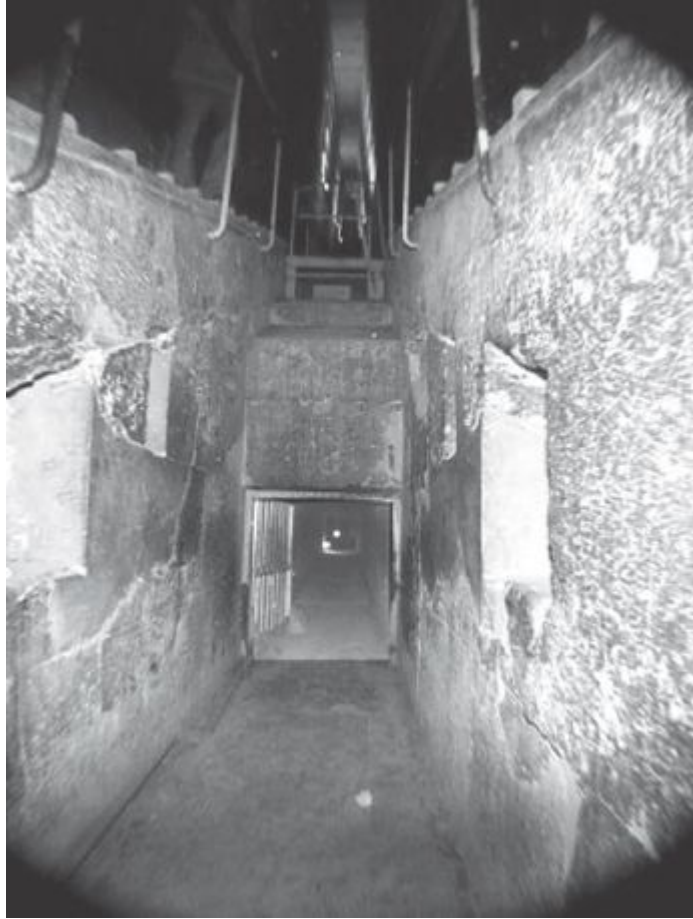
55. Looking toward the entrance to the passageway to the Queen's Chamber
